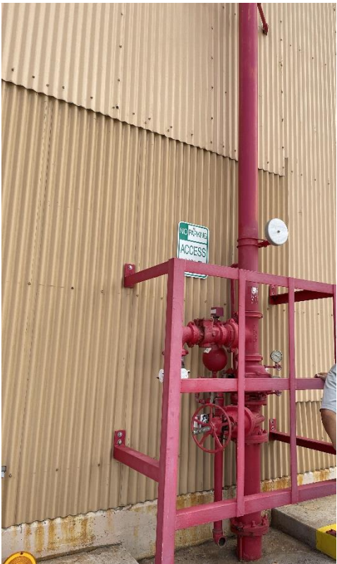
Photo 2: Existing Fire Sprinkler System to be replaced
